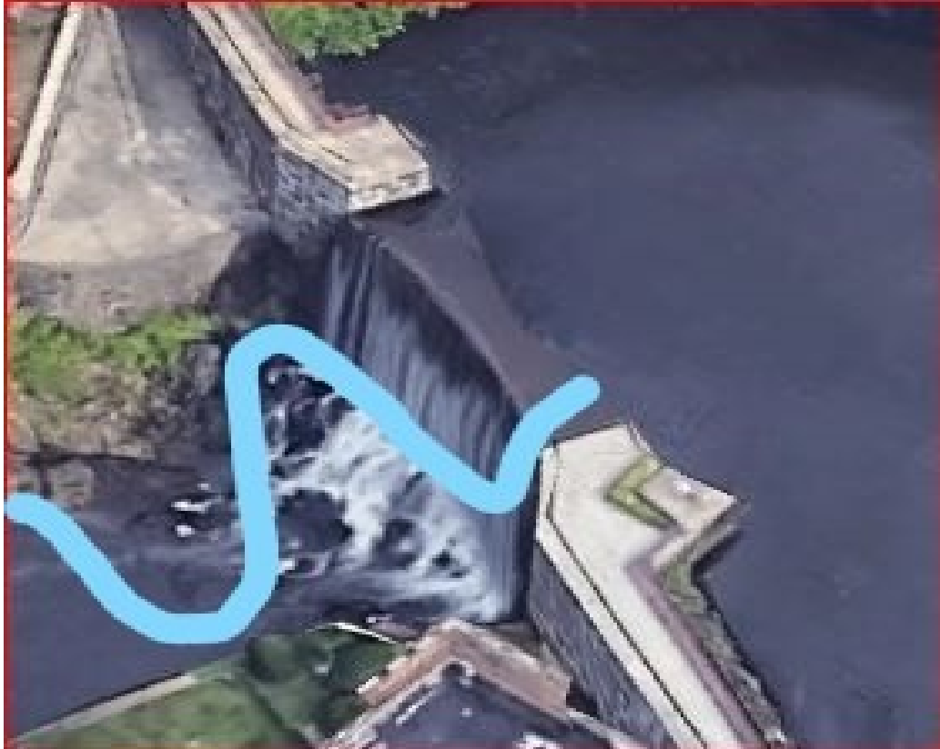
Existing dam with proposed anadromous / diadromous access channel indicated.
