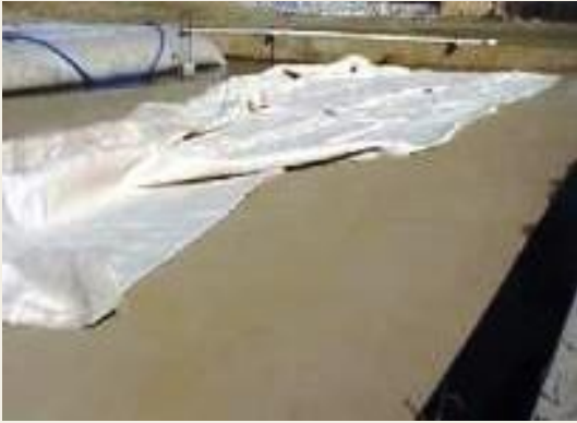
Geotextile dewatering bed
